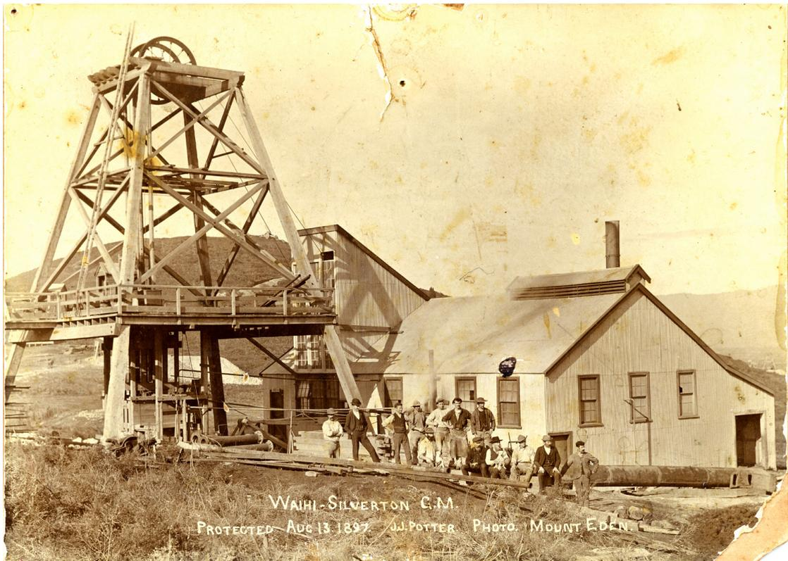
Silverton Shaft 1897. The building housed a wood fired boiler, winding engine, and pumping engine. There are 13 men and two dogs pictured here. Behind the men are squared mine props ready to be taken below. Behind the poppet legs is a mullock tip from the Gladstone shaft, and at the very right of the photograph can be seen (just) the Union No. 2 Shaft poppet. WACMA.
